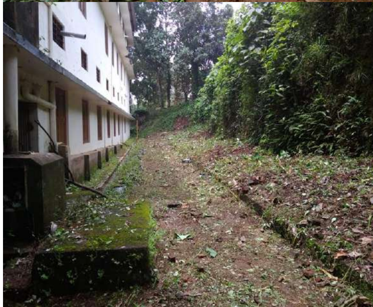
NSS volunteers cleaning the college premises
